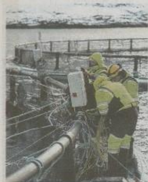
MONTERING: Luselaseren under montering.
