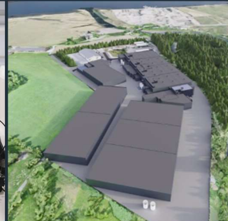
Årdal Aqua (land-based under construction)
